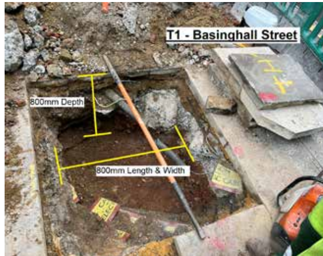
Trial hole excavation
